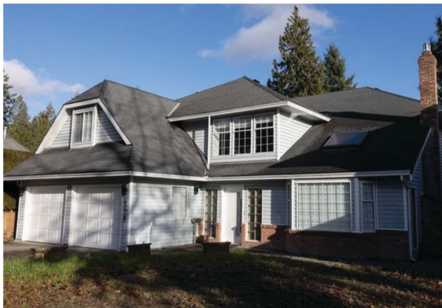
Home in the 6000-block of 133A Street in Surrey. The owners converted the home into four separate rental units but did so without a permit. PHOTO BY JASON PAYNE /PNG
